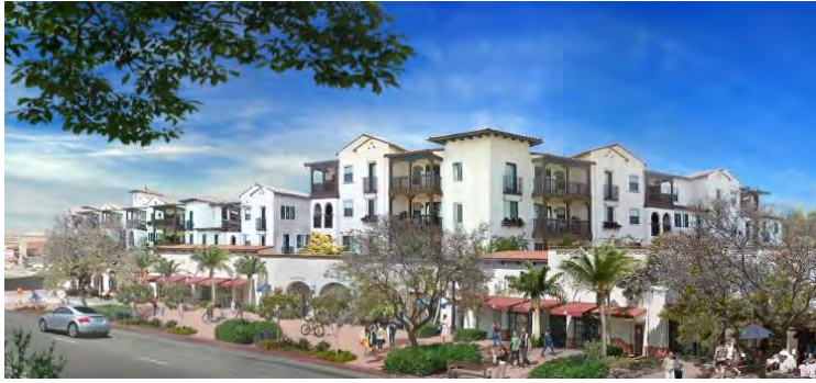
Legado Redondo (Redondo Beach)—3-acre mixed-use project with 115 residential units over 21,539 square feet commercial space 926
